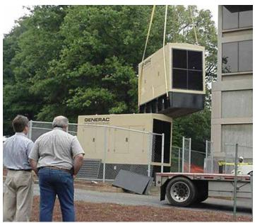
and modular systems comprised of three 500's, four 400's, as well as the 400 / 500 / 600 arrangement that was ultimately chosen. The MPS solution was significantly less expensive than the large unit alone, and the facility now has the added advantage of redundancy. The installation cost was quite reasonable, and all three generators were shipped on a single truck, so that was just another factor that helped us keep our quote as competitive as possible."
